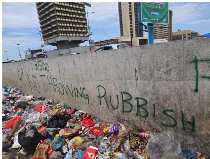
i. Litter on Independence Avenue fly-over bridge
